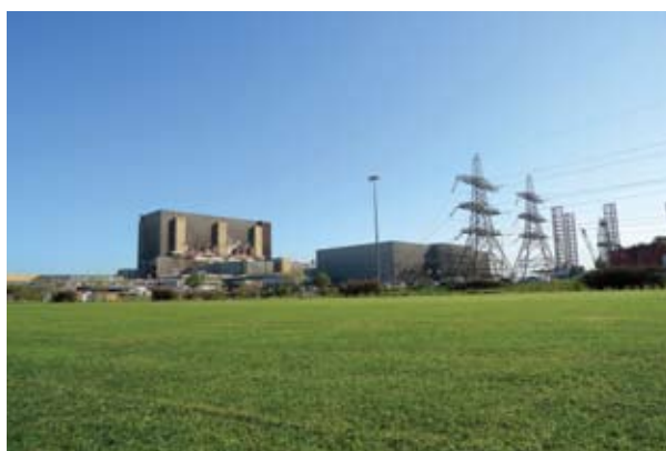
Hartlepool nuclear power station
